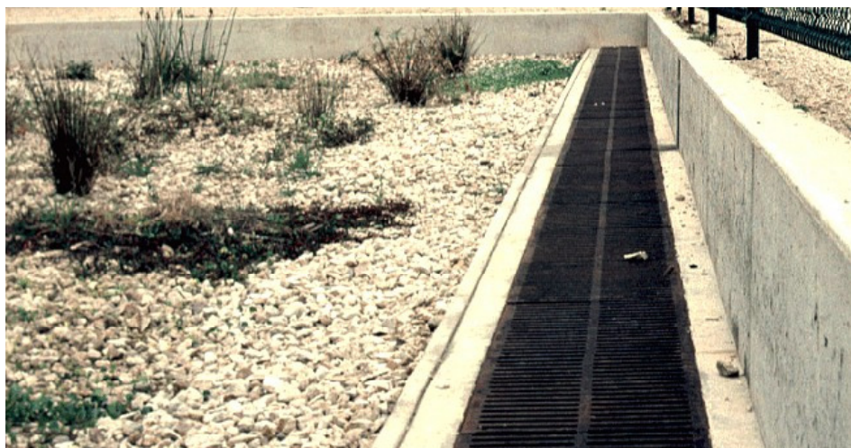
Infiltration bed with overflow grate and pipe
