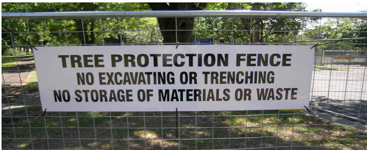
Figure 3: Example of a TPZ warning sign clearly displayed on TPZ fencing
