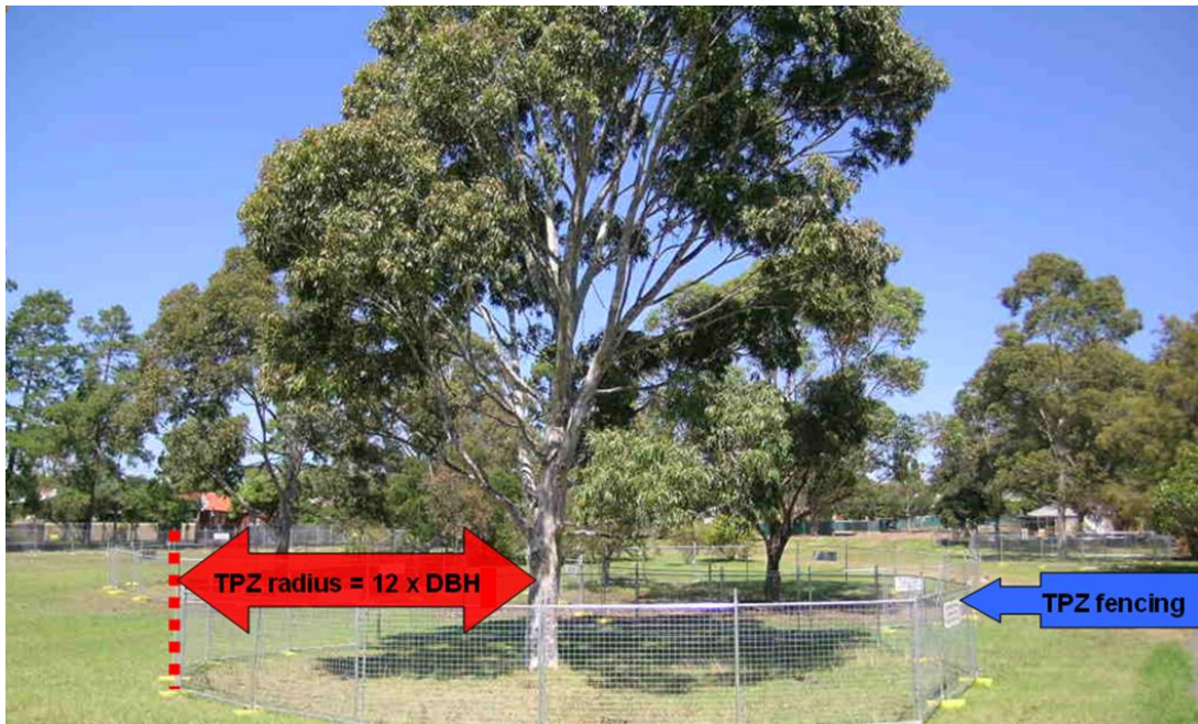
Figure 4: TPZ fencing is erected around retained trees prior to site works.
