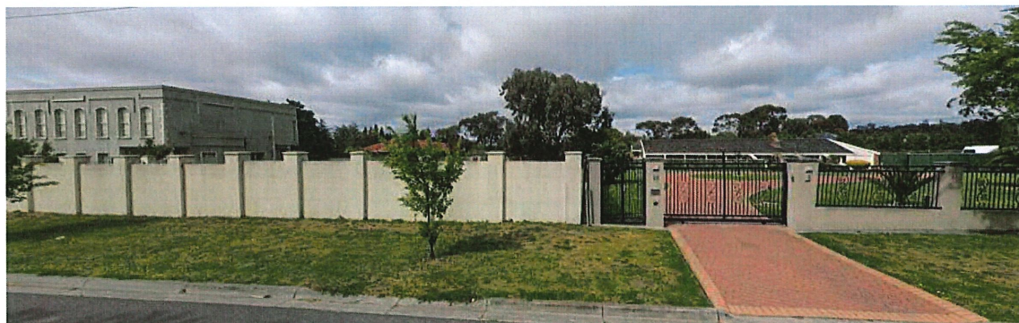
Figure 7 – View Opposite / South of the Site (GoogleMaps)
