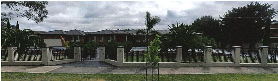
Figure 6 – Abuttal to the West, 22 Elphinstone Boulevard, Greenvale (GoogleMaps)
