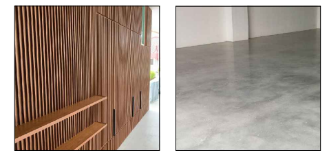
Timber strip Polish concrete
