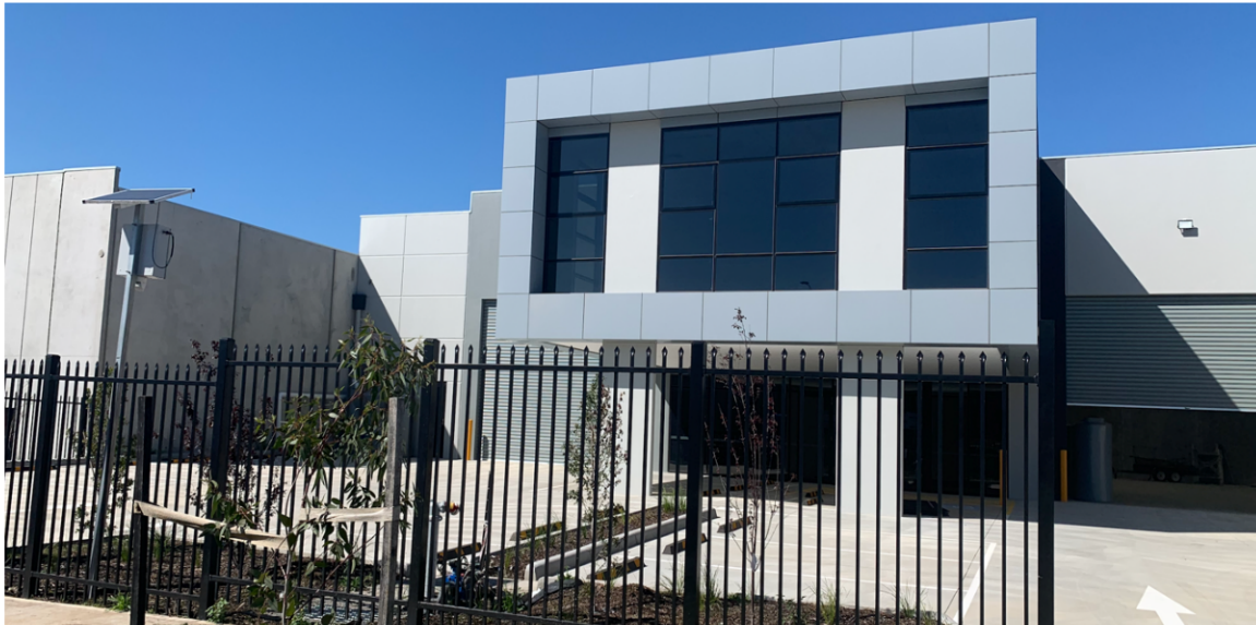
Photo 1 shows view of the warehouse (as constructed)
