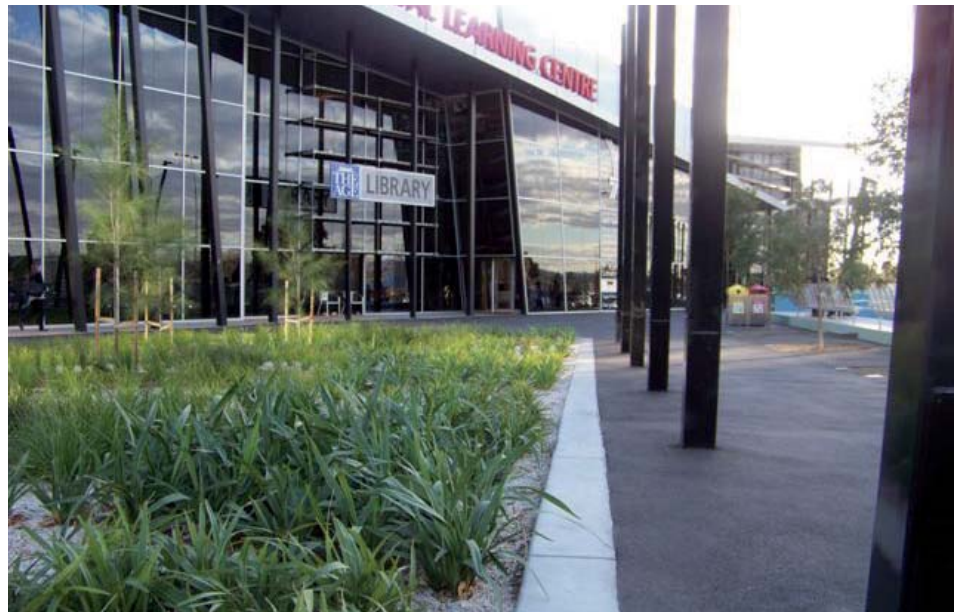
Buffer strip adjacent to paved area
