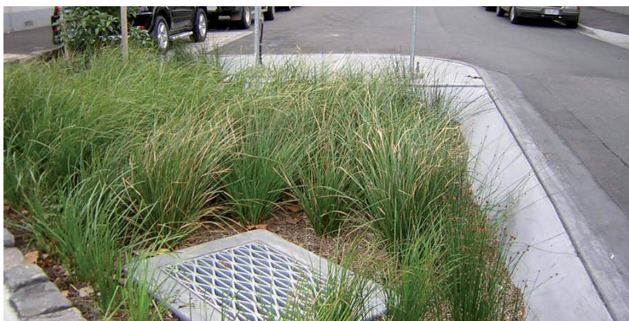
Raingarden alongside a carparking area or internal road
