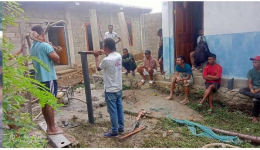
AMYC constructing water bore
