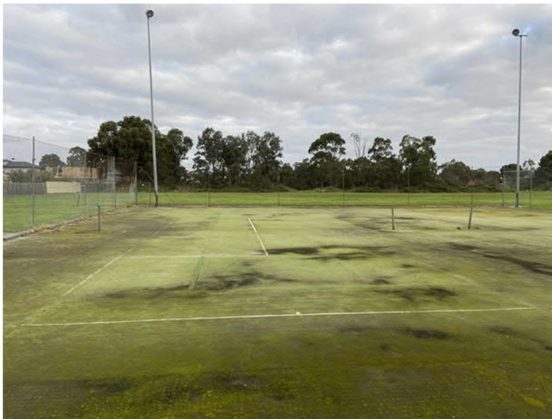
2 courts in very bad condition and very slippery within a fenced area.
